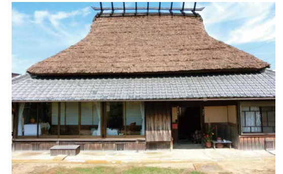
Preservation and utilization of historical structures
